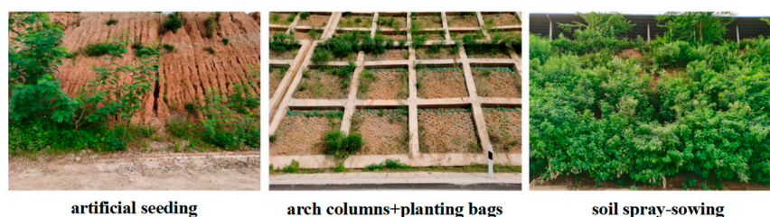
Figure 1. The schematic diagram and effect of artificial seeding, arch columns + planting bags, and soil spray-sowing.
